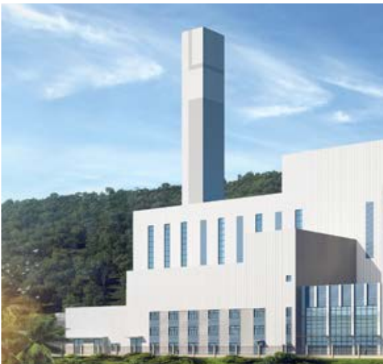
Xiamen WTE Plant Project
