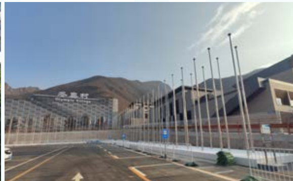
Temporary facilities project in Yanqing Division
