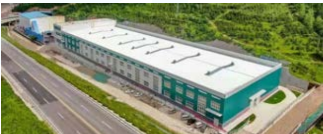
Coal to electricity project of Erdaogou Heat Source Plant in Chongli District, Zhangjiakou City
